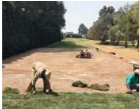
Sodding the enlarged and levelled 5 th tee with cool-season sod.
